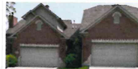
Photo of similar brickwork
